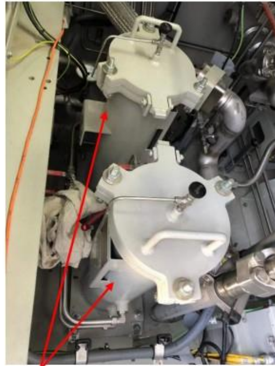
Lubricating oil dual filter
